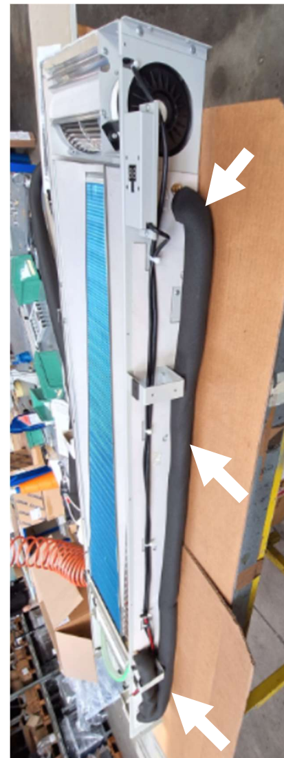
PUT INSULATION IN ALL THE EXTERNAL PIPE
